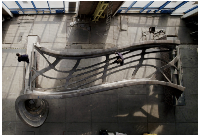
Fig. 1 The MX3D Bridge designed by Joris Laarman Lab, seen from above in MX3D's workshop during production (Courtesy Joris Laarman Lab)
